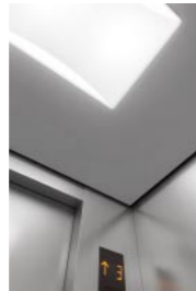
Ceiling: Painted steel sheet (Y033) with a milky white resin lighting cover Lighting: Central lighting
