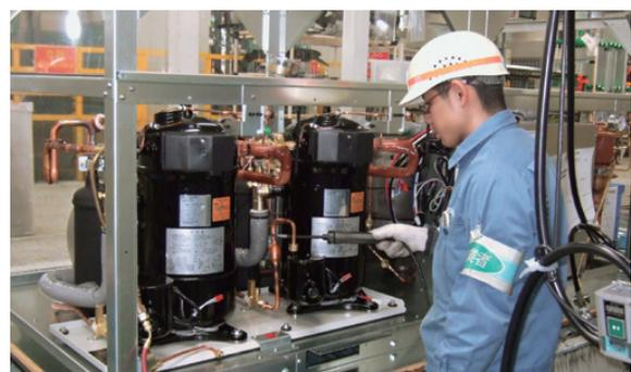
Compressor also developed and manufactured by Mitsubishi Electric\*
